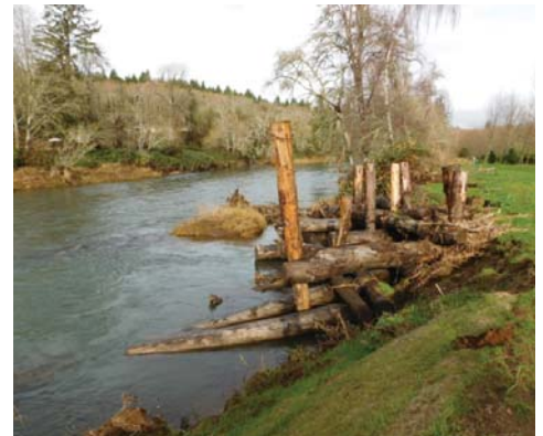
Left: Property before project. Bank erosion was causing Grays River to divert from its channel and migrate toward adjacent open agricultural land. Right: Site after large woody debris jam was installed. This picture was taken after a 25-year flood event.
