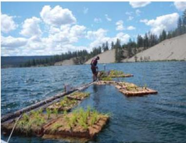
Installed floating wetlands. The logs break waves, which reduces shoreline erosion. Plants will be harvested, removing phosphorus from Lake Spokane. Photo by Charlie Kessler
