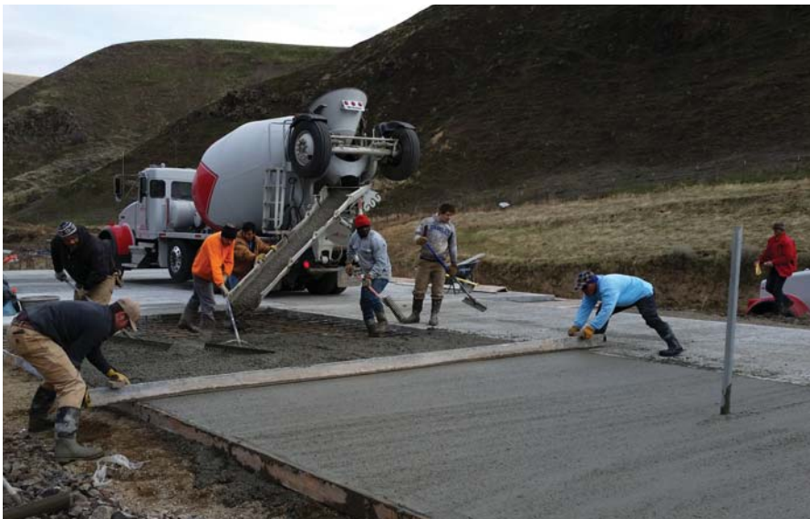
Livestock feeding pads and heavy use areas: Installing stable, non-eroding surfaces in areas frequently used by animals prevents erosion and aids in manure collection. This helps protect water and air quality.
