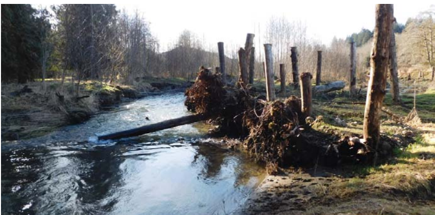
Instream and streambank stabilization structures: Benefits include erosion control and enhanced fish habitat.
