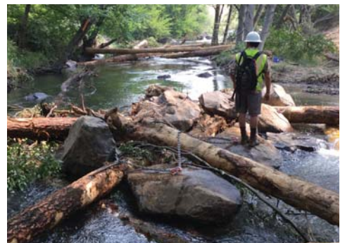
After photo of channel spanning structures. Photo by Justin Pearson
