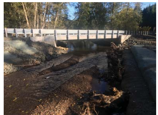
After construction completion. Photo by Tom Kollasch
