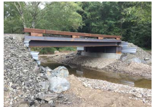
Photos: (Top) Property owner sharing photos of the previous year's flooding of his driveway. (Bottom) One of two new bridges installed.
