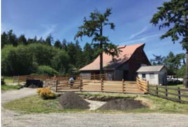
Livestock fencing, manure storage and rain garden under construction.
