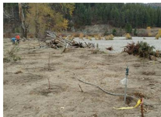
Final stages of the project. Banks are stabilized, woody debris is placed, and buffer is planted.
