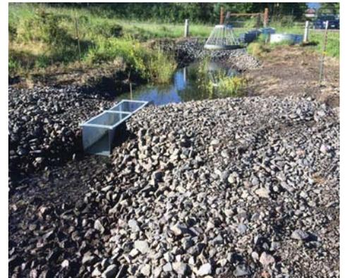
Inlet structure for aquifer recharge trench.
