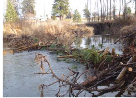
Beaver dam analogue operating under early winter flow conditions.
