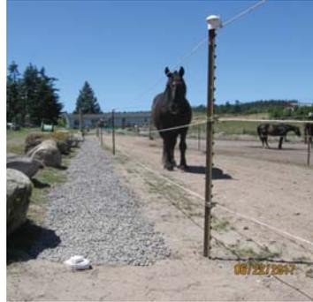
Completed french drain system diverted surface water to existing swale onsite. Photo by Ken Drecksel
