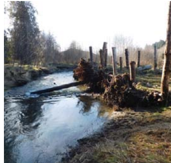
Porous debris jam regulates flow into side channel habitat and creates pool habitat in main stem. Photo by Wahkiakum Conservation District
