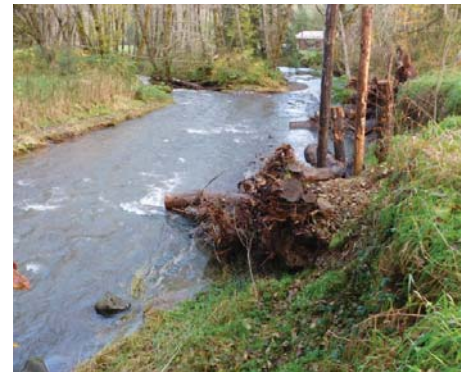
Debris jam deflectors create pool habitat and protect streambank that was once full of junkyard cars. Photo by Wahkiakum Conservation District
