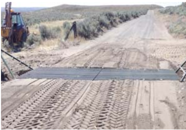
Installed cattle guard to help control animal movement using cost-share.
