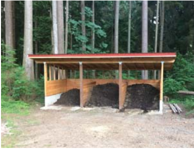
Waste storage facility installation.
