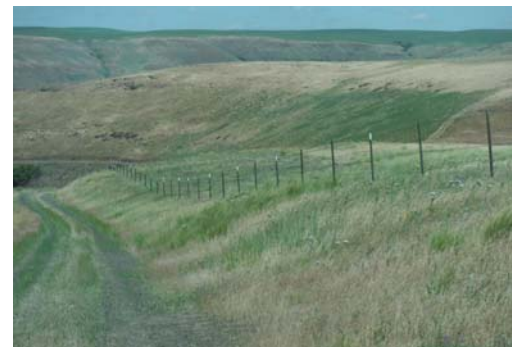
Completed fence along Wawawai grade. Photo by Lance Fredrick
