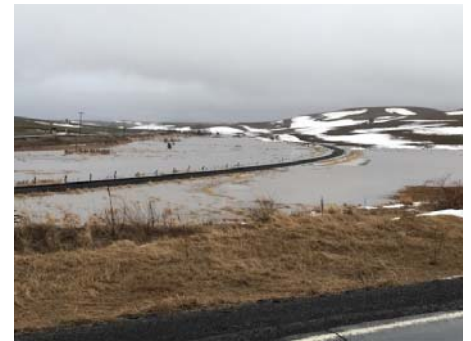
Two streambanks completely submerged, and state railroad surrounded by water and cutting into rail bed.
