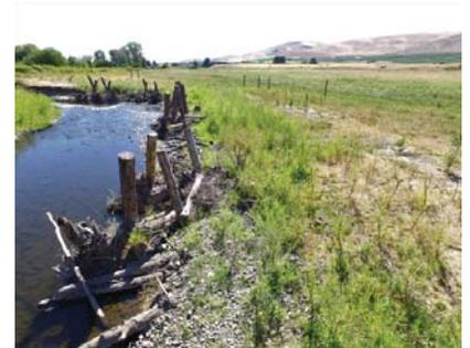
Wood structures with plantings and livestock exclusion fencing. Plantings provide stream shade and improve stream function.
