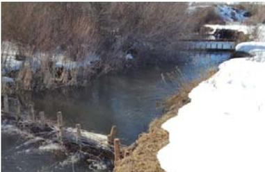
Installed Post Assisted Willow Structures (a.k.a., beaver dam analogs) to assist in floodplain connection portion of Nedrow Project.
