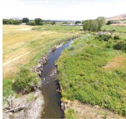
Typical wood structures used in project to stabilize streambank, create habitat, and allow flood water to access floodplain.
