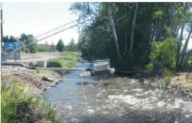
A gravity irrigation diversion was converted to a pump station with fish screen. The passage barrier was removed on Naneum Creek.
