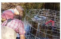
Conservation district staff install a fence and pipe flow device to address flooding from a beaver dam while leaving the dam in place.
