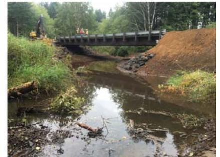
Top: Middle Fork Satsop before project implementation with culvert that restricted fish passage. Bottom: Site after bridge installed allowing for fish passage.
