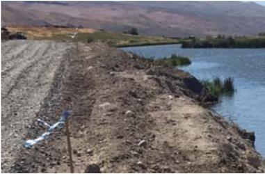
Berming and runoff containment at custom feedlot to protect large fresh water pond from contaminated runoff near Othello. Photo by Lyle Stoltman
