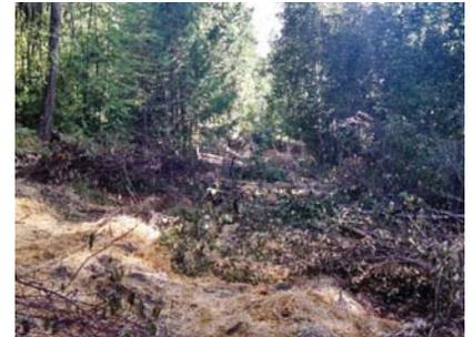
Water is put back into its original bed, and the old road is reclaimed as a riparian buffer.
