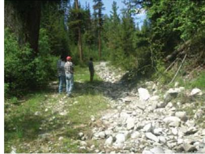
The road bed has become the stream bed. This results in high temperatures, low dissolved oxygen, and siltation.
