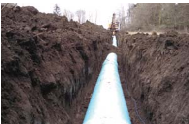
Replaced over three miles of irrigation ditch with pipelines, saving approximately three cubic feet of Dungeness River water per second.
