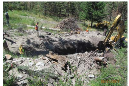
Digging a protective debris diversion while the archaeologist watches for historic artifacts that may need to be documented.
